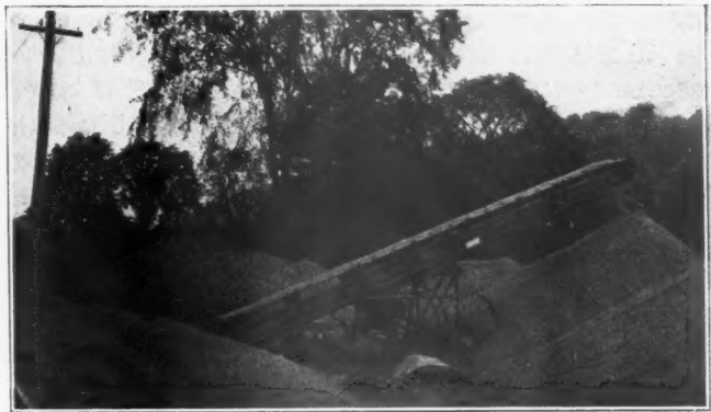
Portable Loader in Storage Piles
